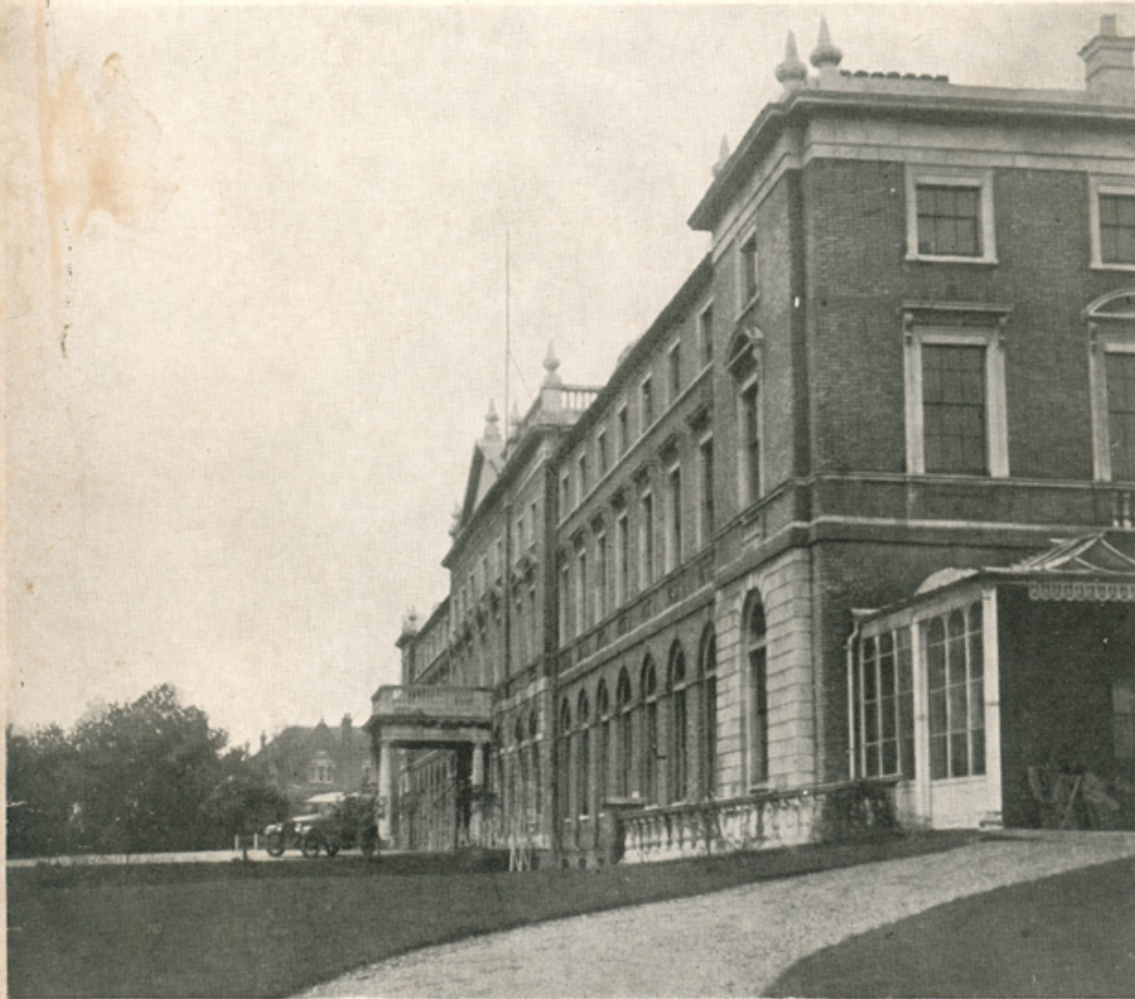
MAIN ENTRANCE FROM SOUTH.
